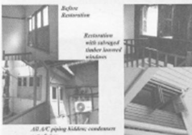
All A/C piping hidden; condensate out of view
