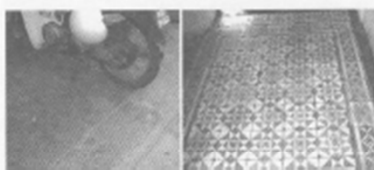
5-foot way, excavated and refilled with salvaged traditional geometric tiles/granite borders retained
