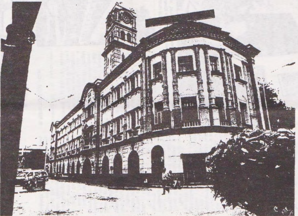
The building that did it all ... the former railway building, now Wisma Kastam, was said to have disrupted the excellent feng shui of Kong Hock Keong.
