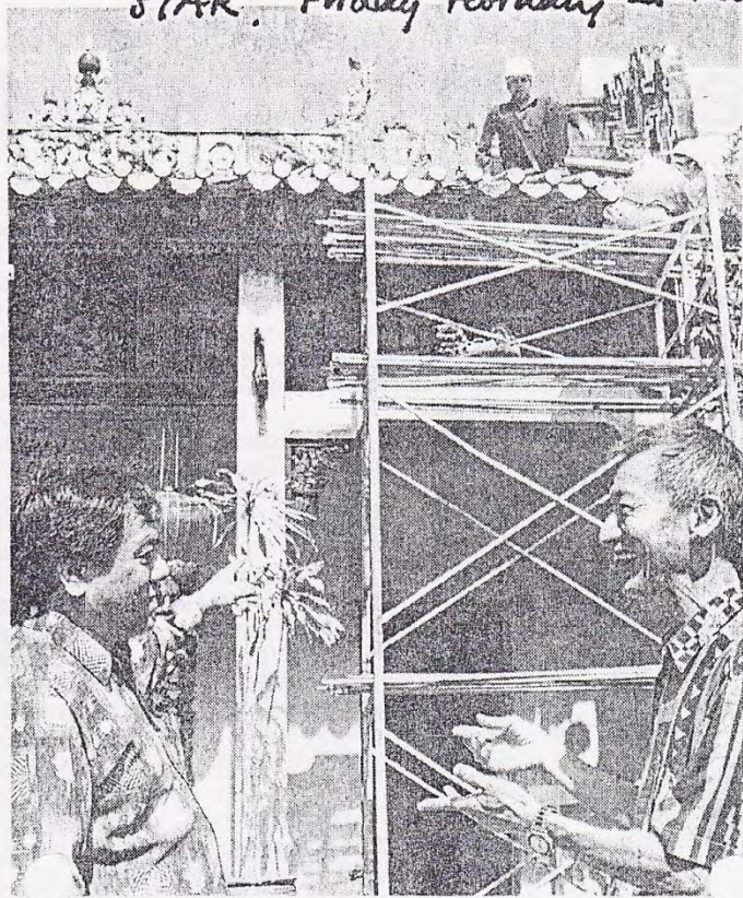
HERITAGE TREASURE... Teoh (left) discussing the restoration project with Dr Choong while two craftsmen from Xiamen inspect the roof.
