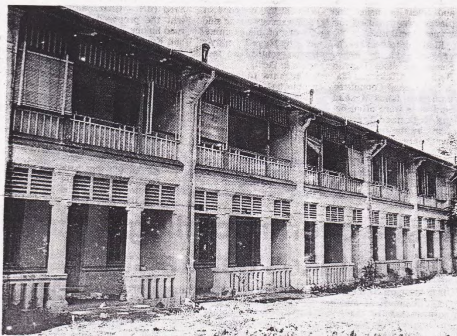
GOVT QUARTERS ... to be converted into 96 hotel rooms — Starpic by LEONG HON HYEAN
