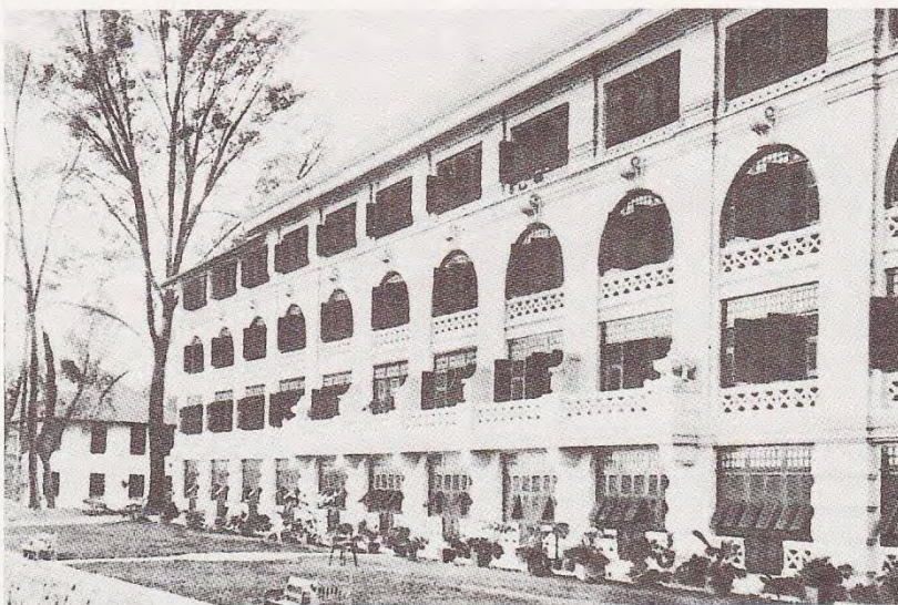
EASTERN AND ORIENTAL HOTEL, PENANG, THE NEW WING.
